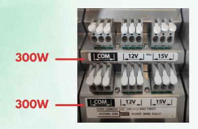
Please ensure that you do not exceed the capacity of the transformer as it can lead to overheating and overload, potentially reducing its lifespan. It is recommended to utilize only up to 85% of the transformer's capacity.
